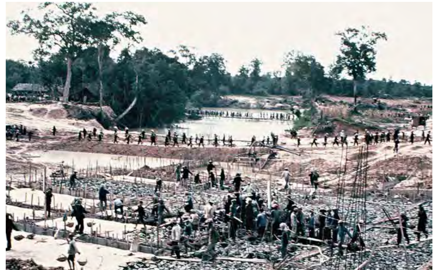
Irrigation dam construction on the road north in 1978. Photo by Gunnar Bergstrom. For fourteen days in 1978, Bergstrom and other members of the Swedish Cambodian Friendship Association undertook a “public relations” tour choreographed by the Khmer Rouge, whose intention was to use the Swedes to rally support for the Khmer Rouge from abroad—particularly from other communist countries. A collection of Mr. Bergstrom’s photos during the trip was published in a book titled, “Living Hell.” (Gunnar Bergstrom/ Documentation Center of Cambodia Archives)
